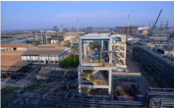
Hydrochloric Acid Plant
