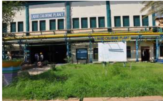
Liquid Chlorine Plant
